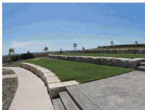
Replace timber edges with new sandstone logs terrace walls
