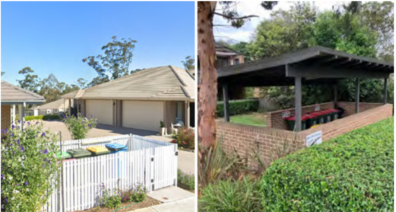
Figure 4: Example of communal waste storage area as part of independent living unit complex (Seniors Housing Design Guide, NSW Planning and Environment)
