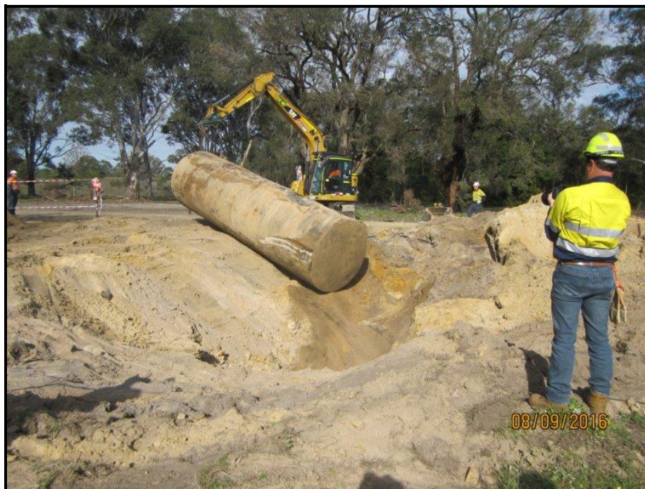
Photo 6: Photograph of the UST being removed from the ground, facing south.
