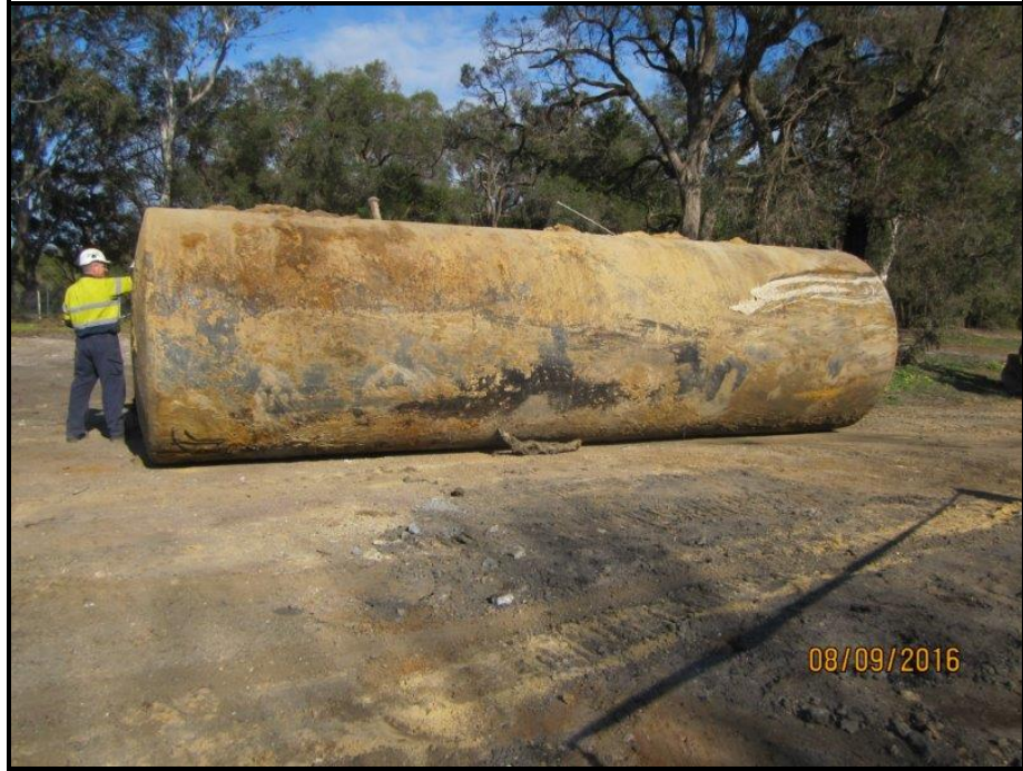
Photo 7: Photograph of the UST showing size and condition, facing south.
