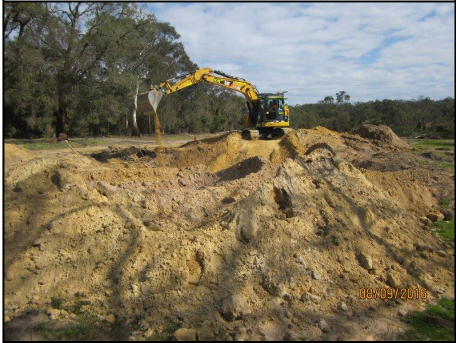
Photo 9: Photograph showing the excavation of packing sands, facing west.
