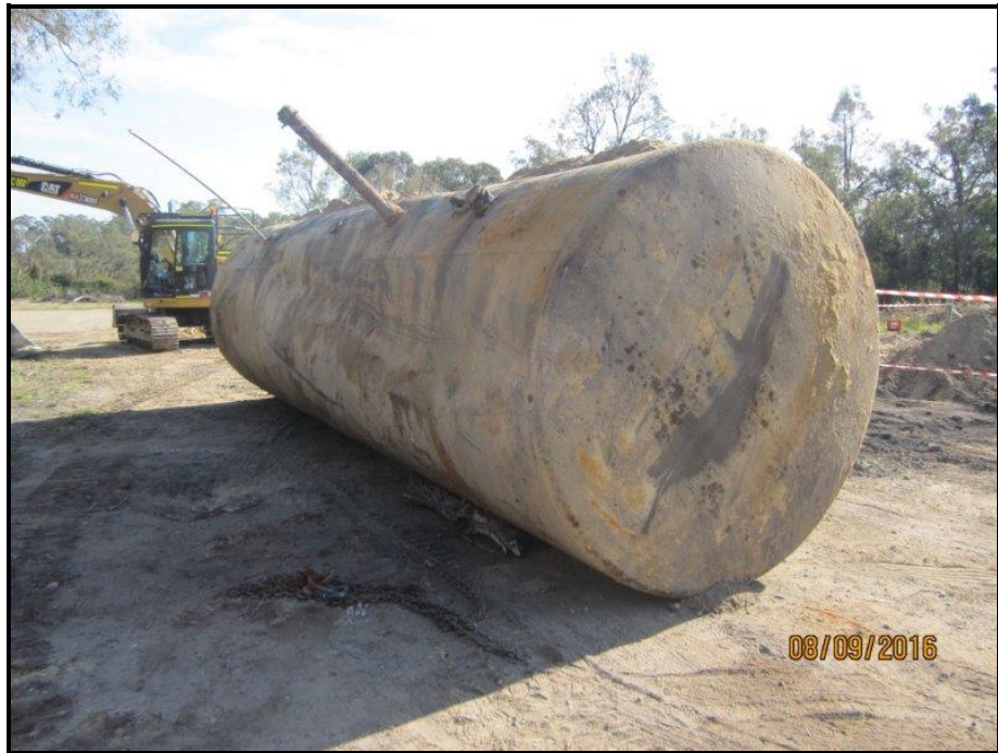
Photo 8: Photograph of the UST showing size and condition, facing north west.
