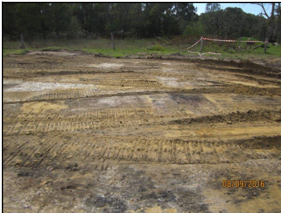
Photo 12: Photograph of backfilled and track rolled UST excavation, facing north.
