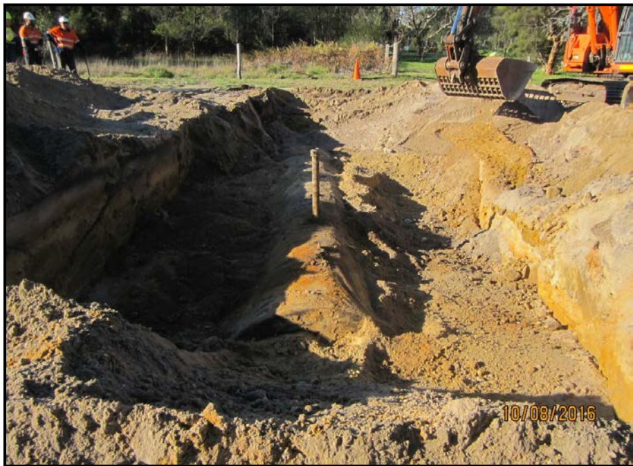
Photo 4: Photograph of the uncovered UST, facing north.
