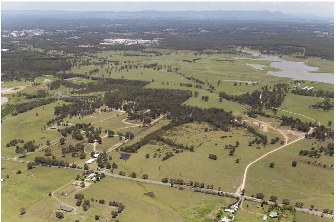
Figure 6 –North eastern extent of the Hydro Site, with Cessnock Road on the foreground, proposed residential development area in the mid ground and Smelter in the background.
