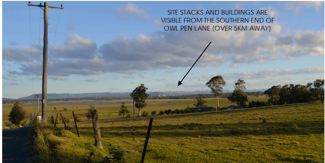
Figure 2-21 View Toward the Site from Owl Pen Lane, Bishops Bridge
