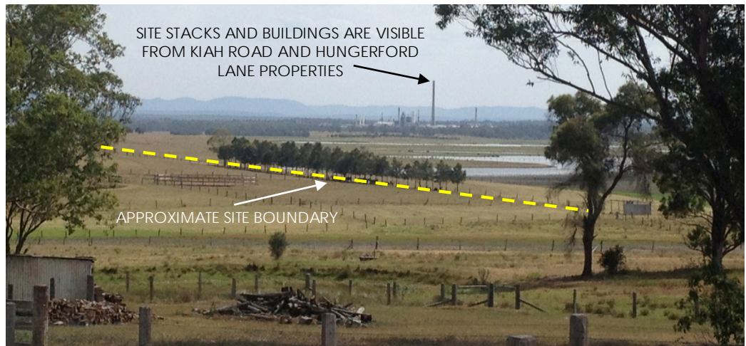
Figure 2-20 View of the Site from Kiah Road
