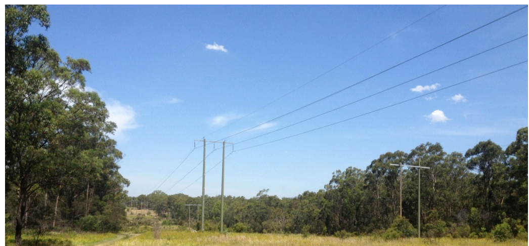
Figure 2-6 View of forest and transmission line clearing
