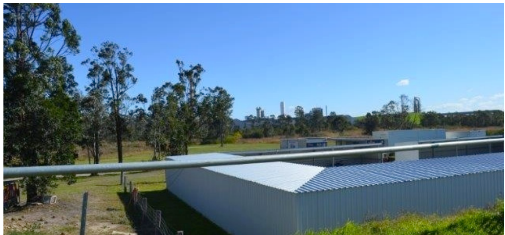
Figure 2-8 View of plant from Kurri Kurri Speedway
