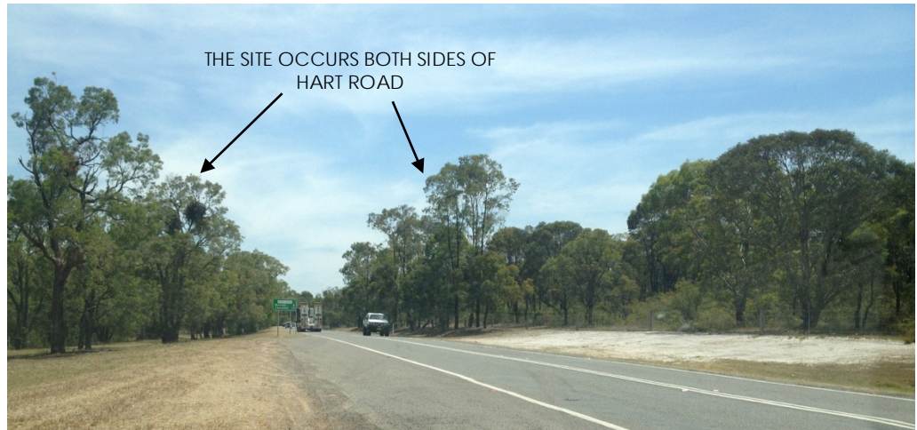
Figure 2-10 Southwestern view of Hart Road
