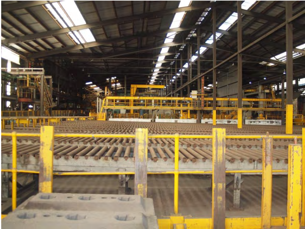
Plate 9 Anode Rod Building - interior
