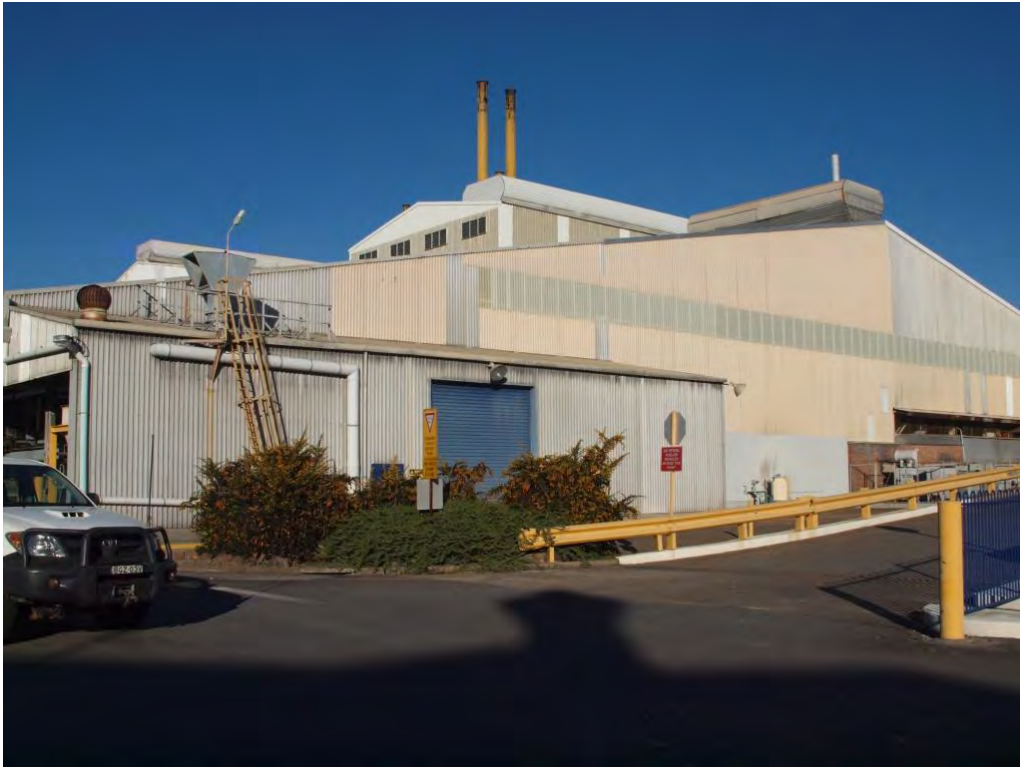
Plate 3 Looking south west to Cast House
