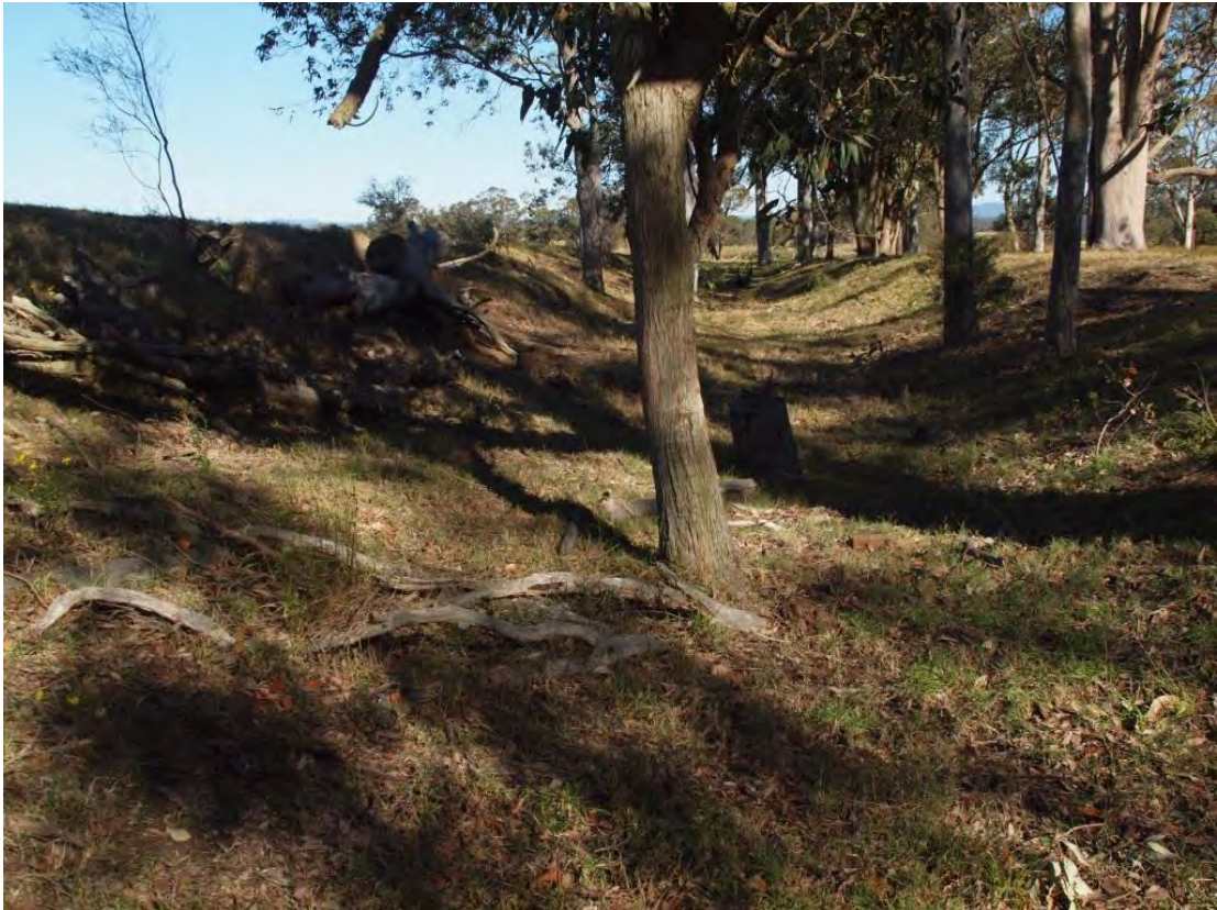
Plate 37 South Maitland Railway cutting deviation - Glen Greta (Glen Main) Colliery subsidence (looking south)
