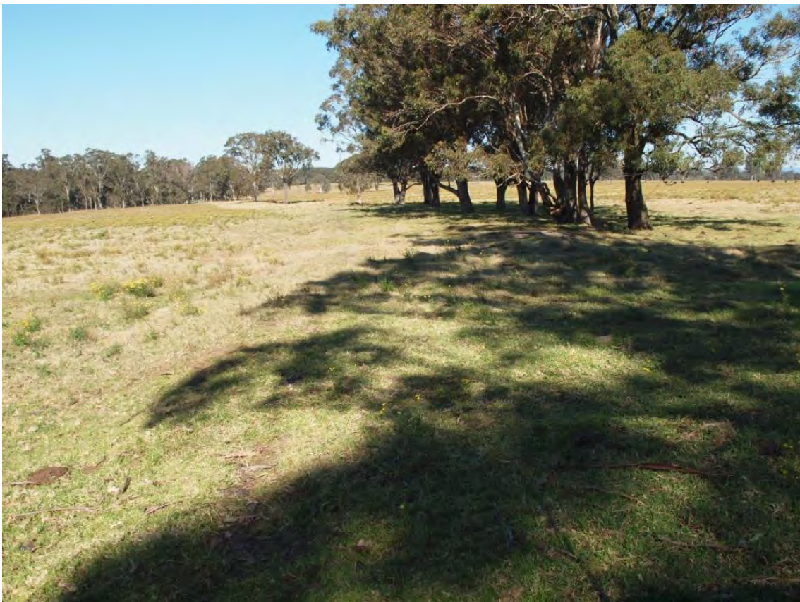
Plate 32 Stanford Railway – looking south east along embankment
