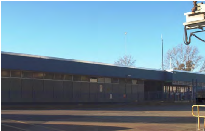
Plate 22 Ancillary building – administration (looking south east)
