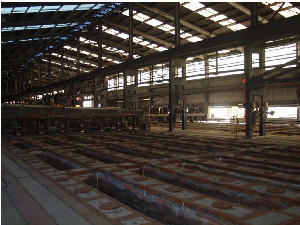
Plate 6 Carbon Plant – interior
