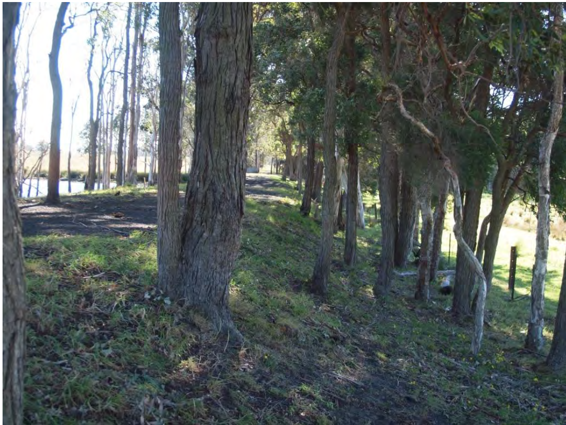
Plate 33 Stanford Railway– looking north along embankment
