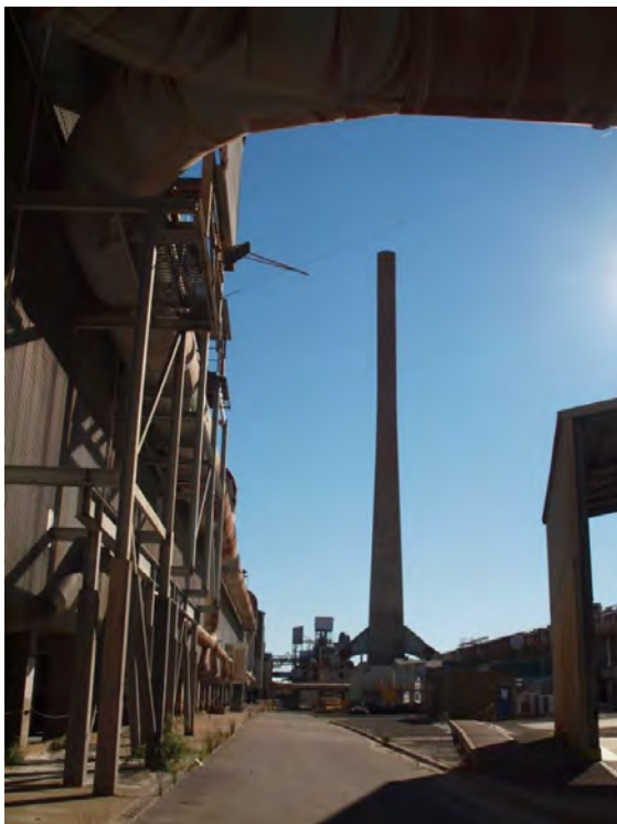
Plate 20 Looking north to chimney
