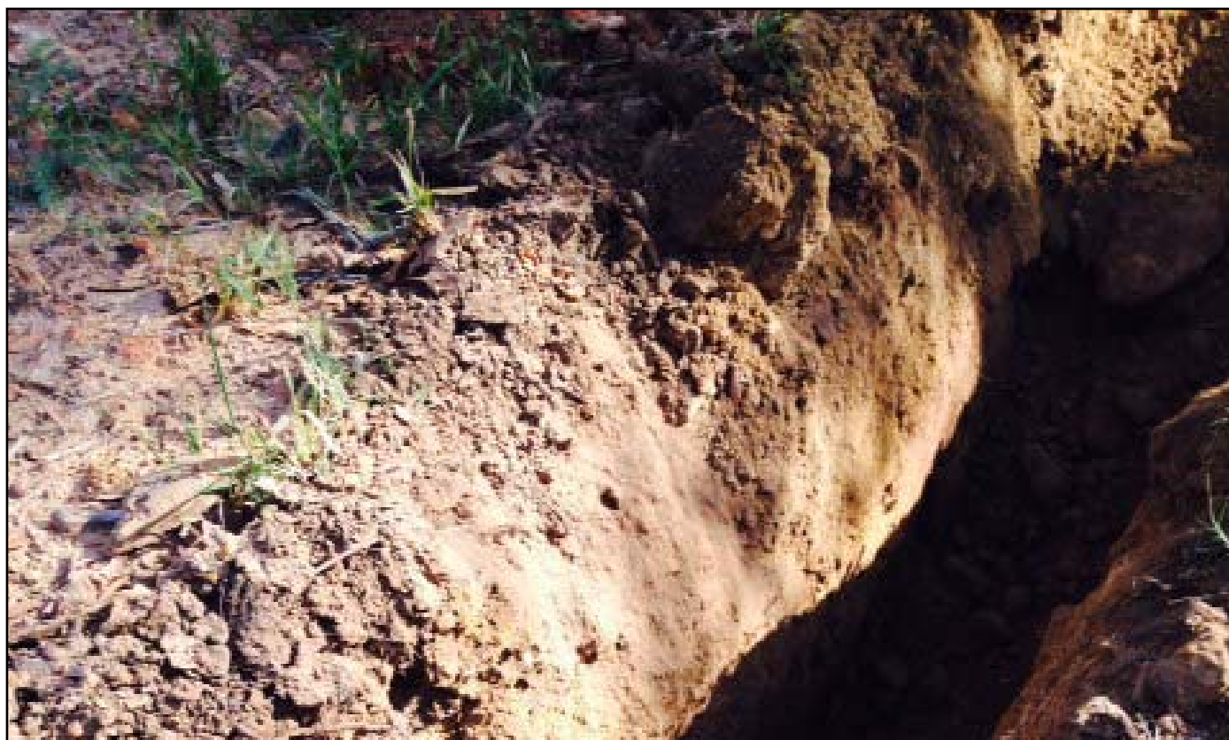
Plate 3: Excavation in stockpile showing subsurface soils
