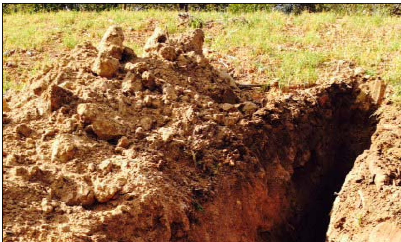
Plate 4: Excavation in stockpile showing spoil
