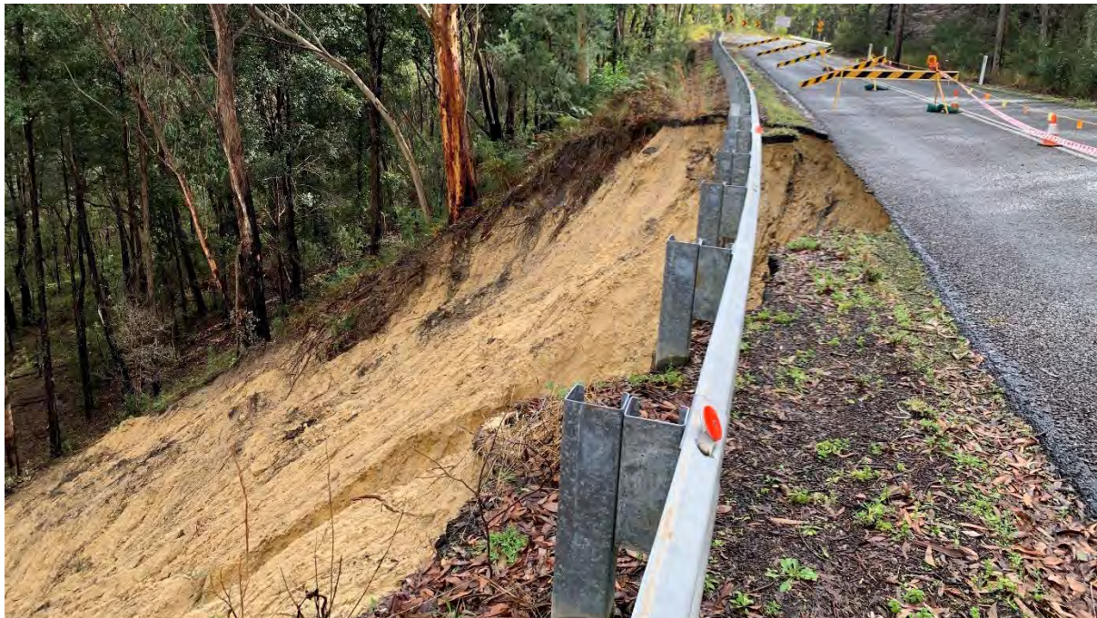
Plate 3. View north at severe landslip affecting the northern portion of the Project Area. (Source: Heritage Now 2022)
