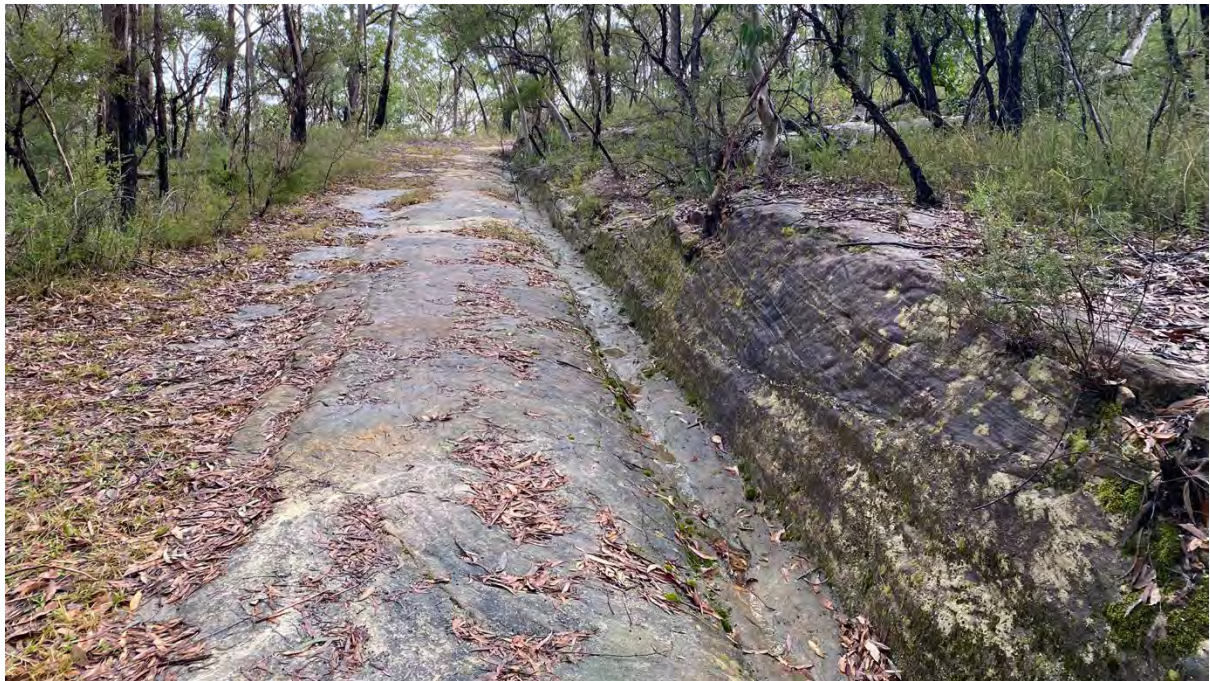
Plate 7. Former road alignment with road pavement cut into bedrock, and associated rock-cut drain (outside of Project Area) (Source: Heritage Now 2022)
