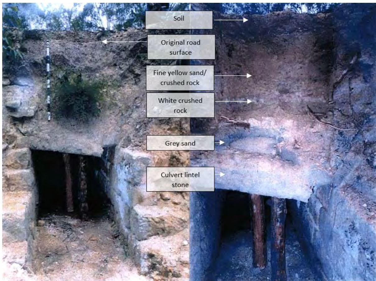
Figure 12. Before (left) and after (right) photographs of the excavation above the culvert. (Source: Roberts, Bucketty Culvert Reconstruction Report , p. 11). Interpretation and labelling of deposits is based on general descriptions provided in the report.
