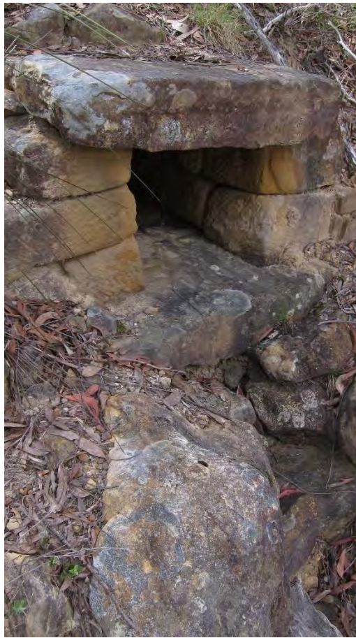
Plate 11. Sandstone box culvert downstream discharge below 1830 alignment of Great North Road, view east (outside of Project Area). (Source: Heritage Now 2023)
