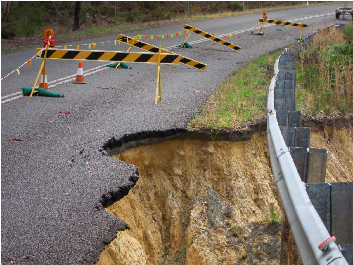
Plate 26. Section of pavement construction exposed by the landslide. (Source: Heritage Now 2022)
