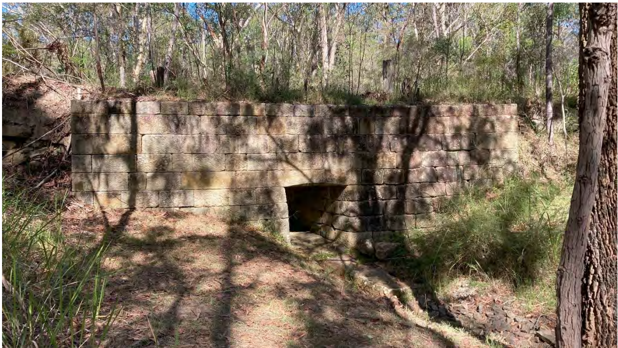
Plate 4. Sandstone masonry culvert with reconstructed wing walls, view south (Source: Heritage Now 2022). Note the culvert runs below the current road.
