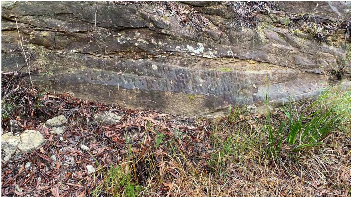
Plate 24. Pick marks on sandstone cutting within northern portion of Project Area (detail) (Source: Heritage Now 2022)
