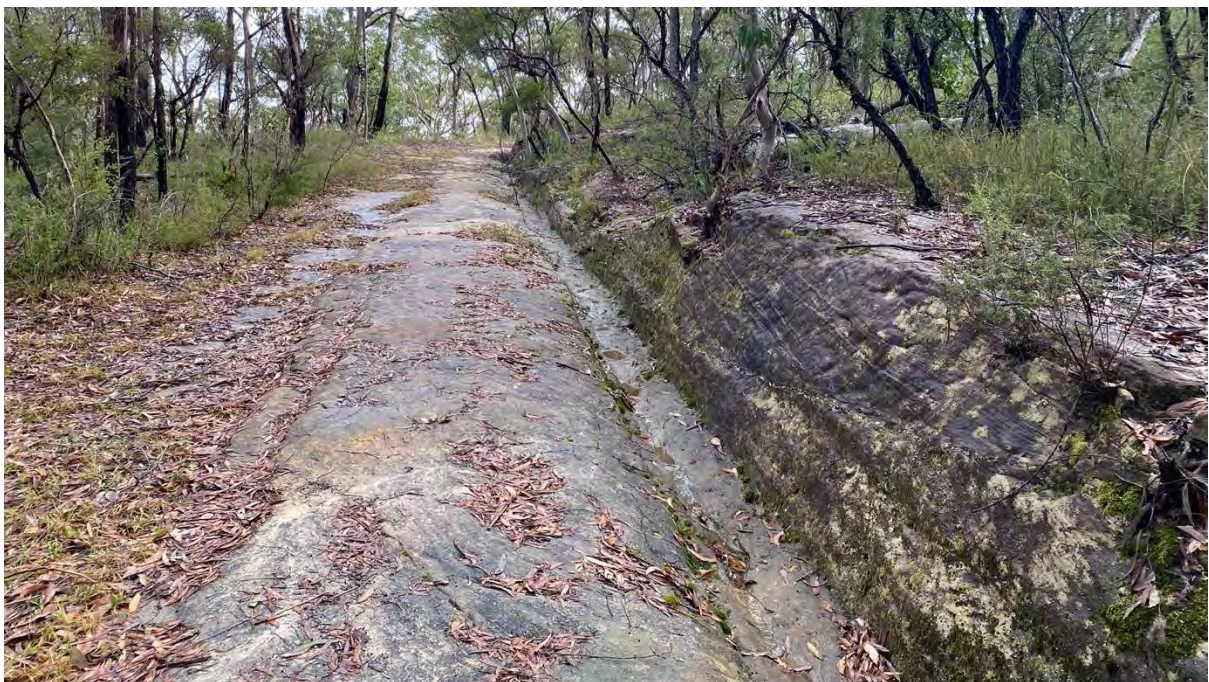
Plate 8. Former road alignment through sandstone cutting and associated rock-cut drain, view north-west (outside of Project Area). (Source: Heritage Now 2022)
