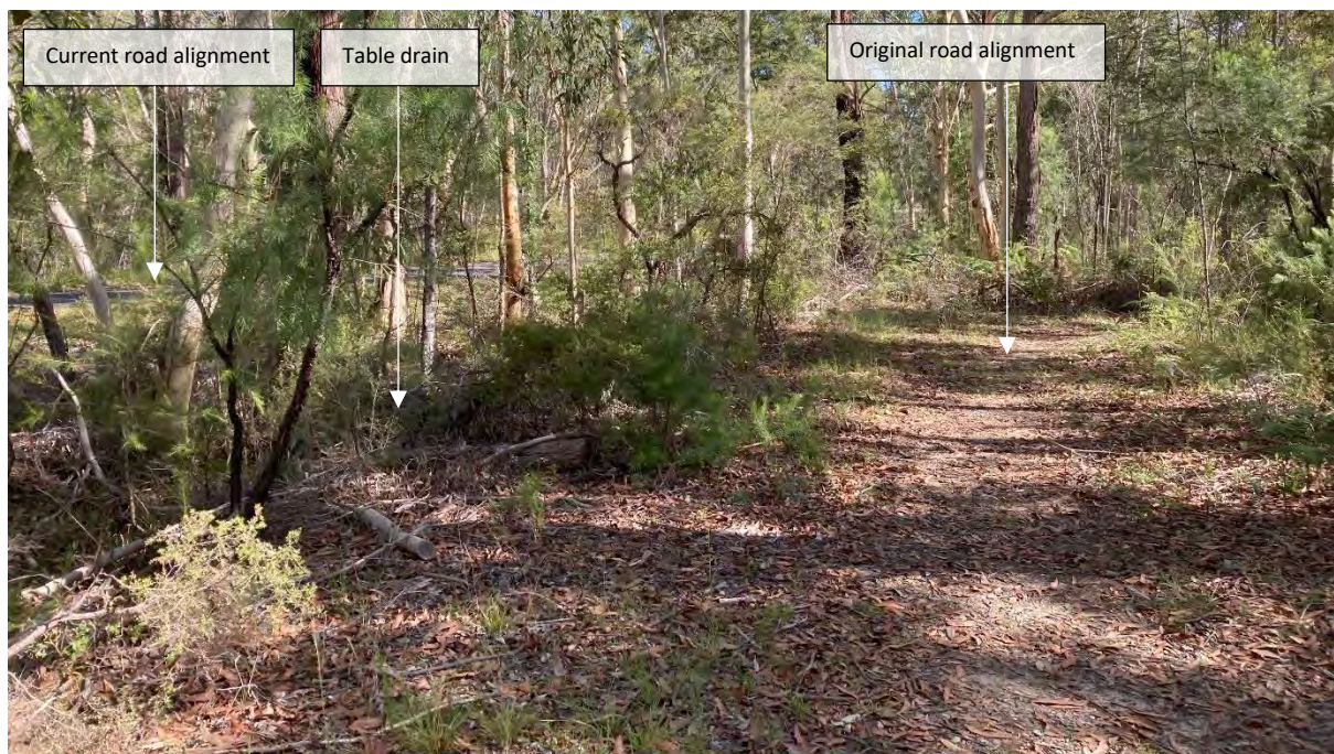
Plate 5. Original 1830 alignment of Great North Road [Road pavement 1] and table drain (adjacent to the Project Area), view west (Source: Heritage Now 2022).
