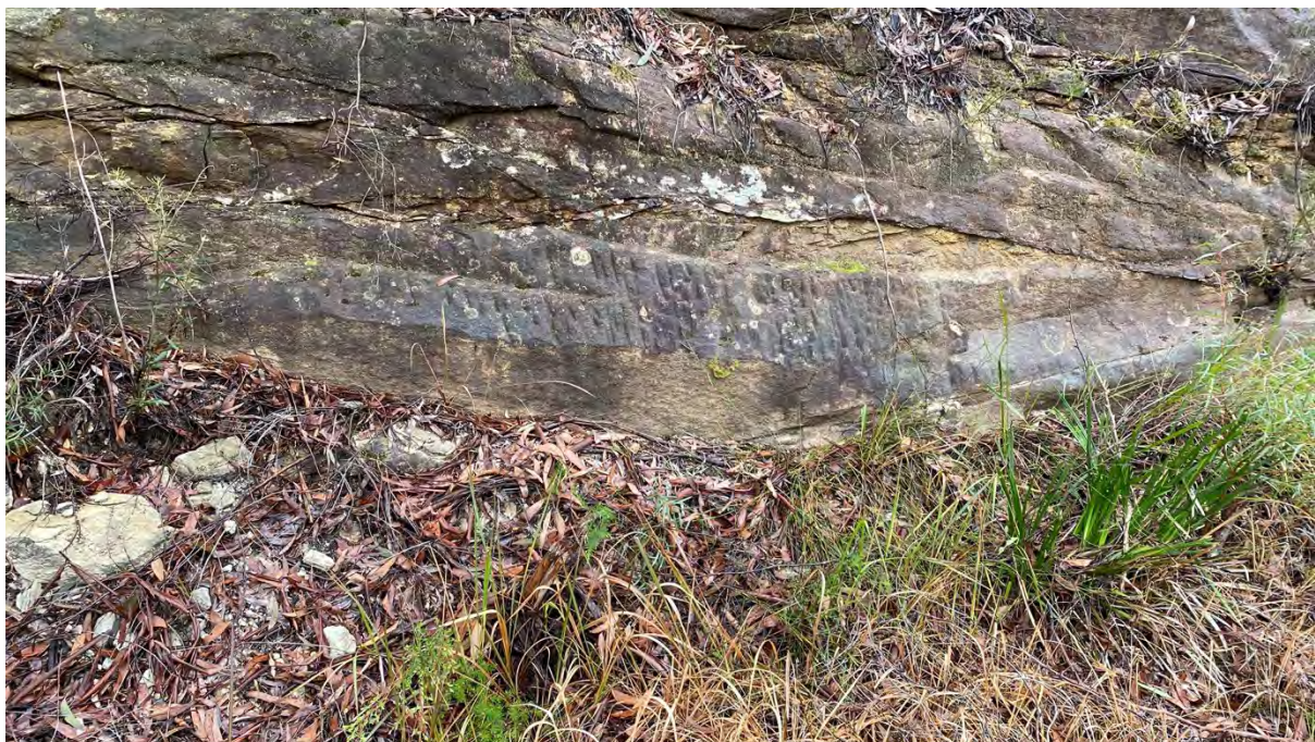
Plate 10. Pick marks on sandstone cutting within northern portion of Project Area (Source: Heritage Now 2022)
