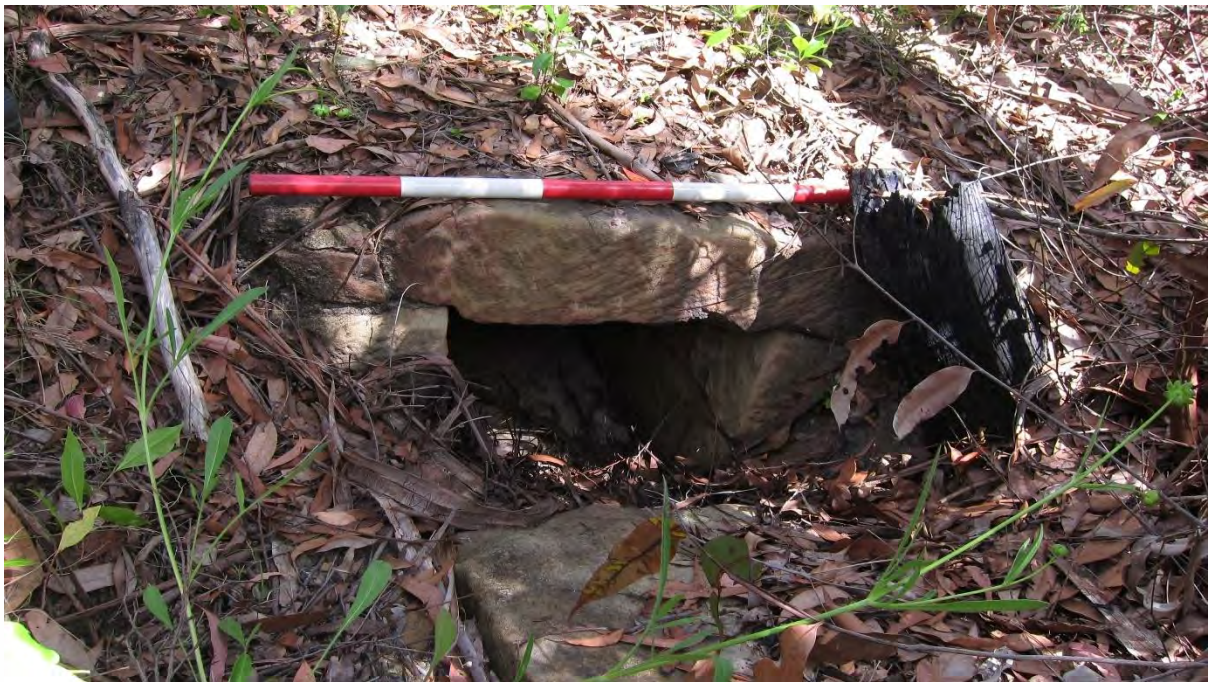
Plate 10. Sandstone box culvert upstream entry above 1830 alignment of Great North Road, view west (outside of Project Area). (Source: Heritage Now 2022)
