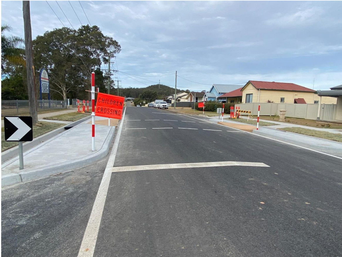
Figure 4 – Anderson Avenue Paxton – Post-works Photograph
