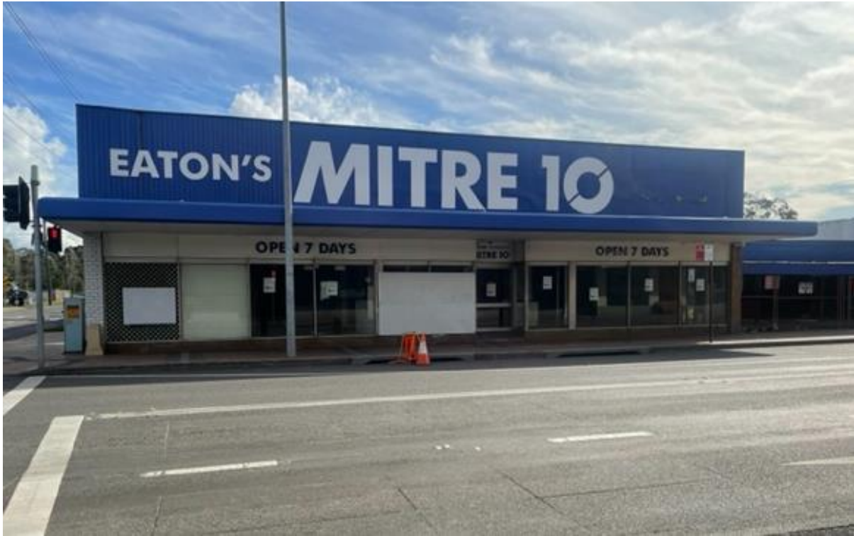
Figure 2: Site from Vincent Street frontage
