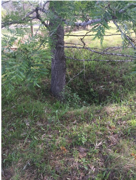
Pothole formation near a tree on the northwestern side of the site
