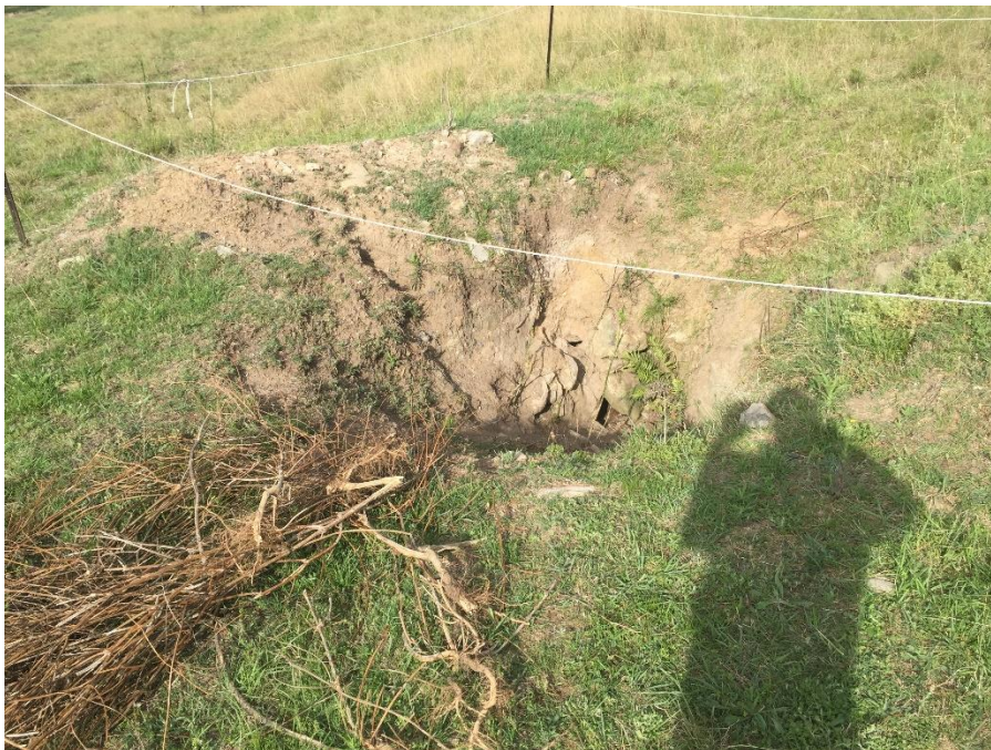
Pothole formation on the northwestern side of the site. Note the area being roped off.
