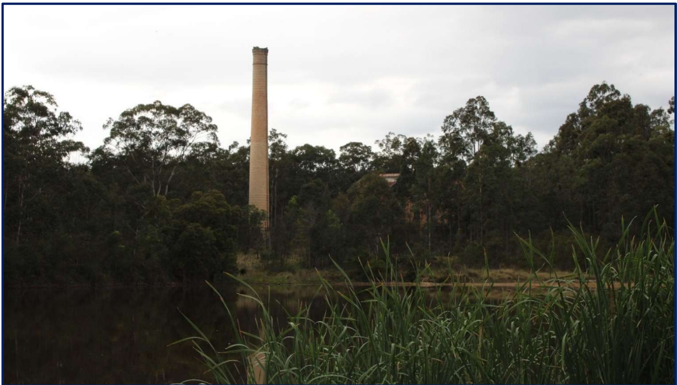
Plate 2: Abernethy Dam and former colliery infrastructure
