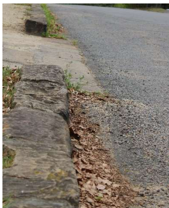
Plate 6: Sandstone kerb and guttering
