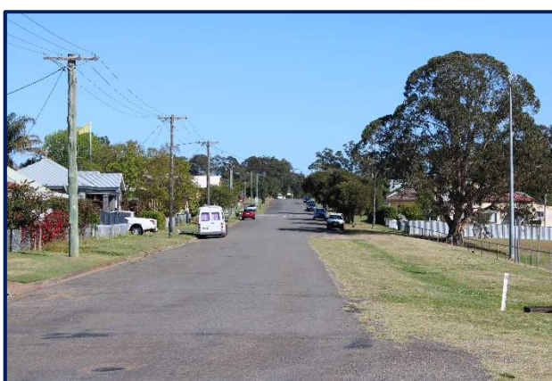
Plate 1: Views along Stanford Street (left and top) to the west and north, Local Streetscape view (bottom)
