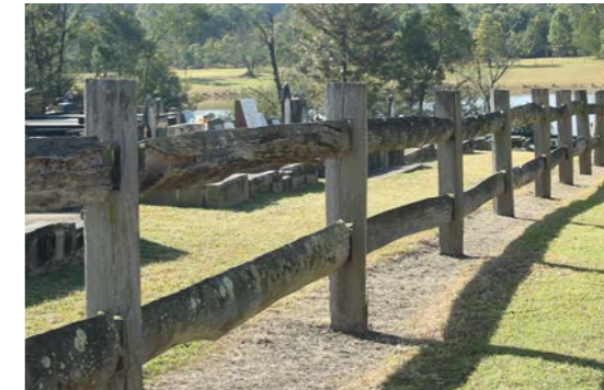
Example of traditional rural timber fence at Wollombi
