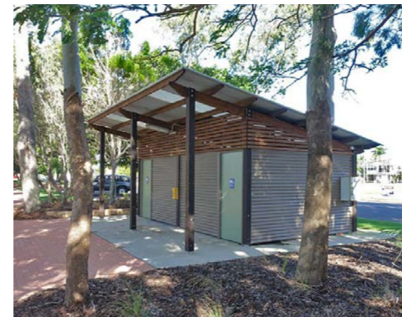
Example of freestanding toilet structure
