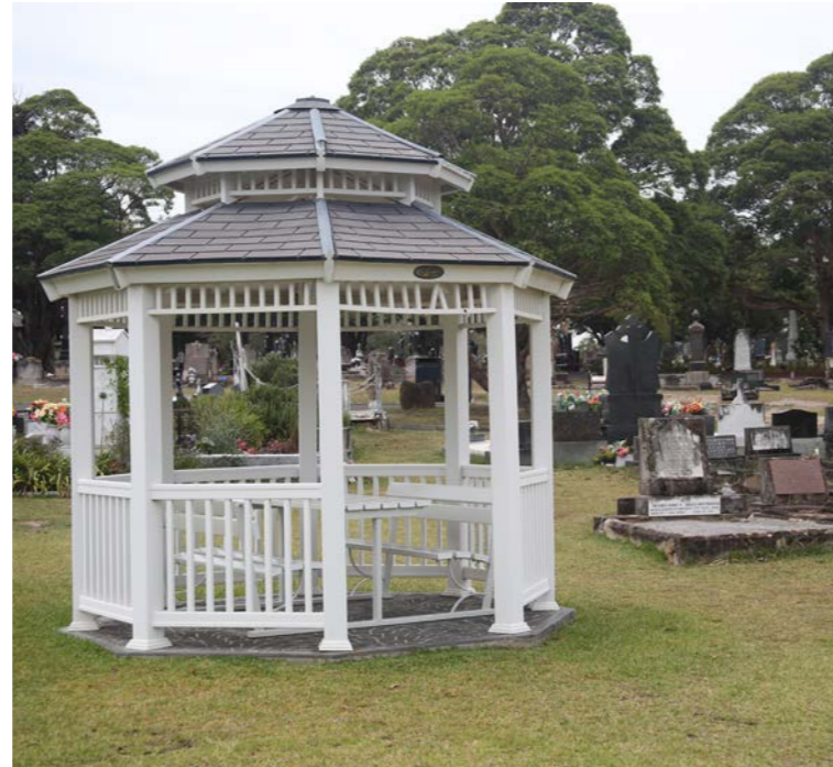
Example of timber shade structure in Woronora, NSW
