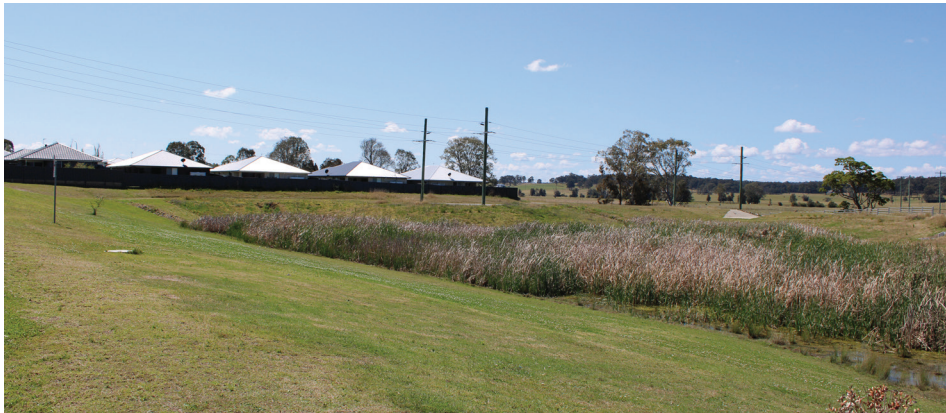
Plate 20: Stormwater Management Infrastructure Example
