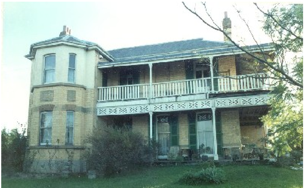
'Dunoon' two-storey Victorian House, Buchanan Road, Buchanan, built in 1883.
