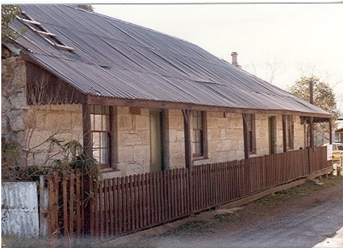
The construction method used for the cottage is of scientific interest as it is an example of a cheap house erected during the early development of a rural New South Wales town during the 1830's. It is known as Caroline Chisholm Cottage, No.3 Mill Street, East Maitland.
