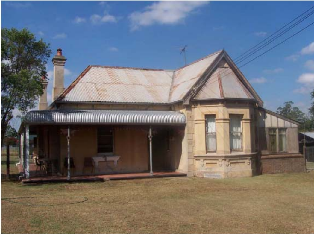
An example of a Victorian brick cottage with galvanised iron roof and bull-nosed verandah roof.
