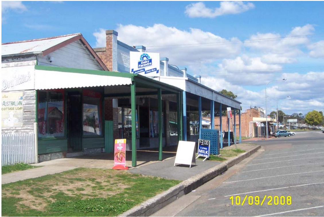
Original shopfronts add variety and richness to the streetscape and shall be preserved.
