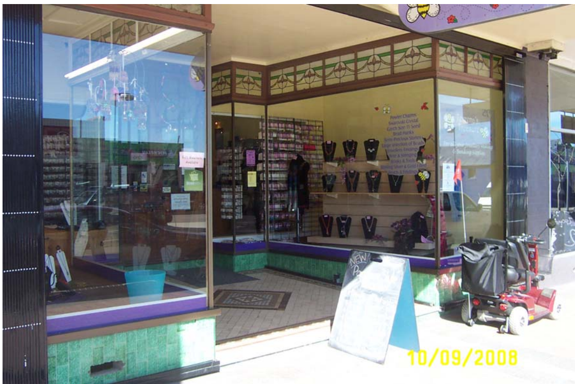
Early shopfronts are characterised by recessed entries, display areas and the use of tiles, stained glass and colour.
