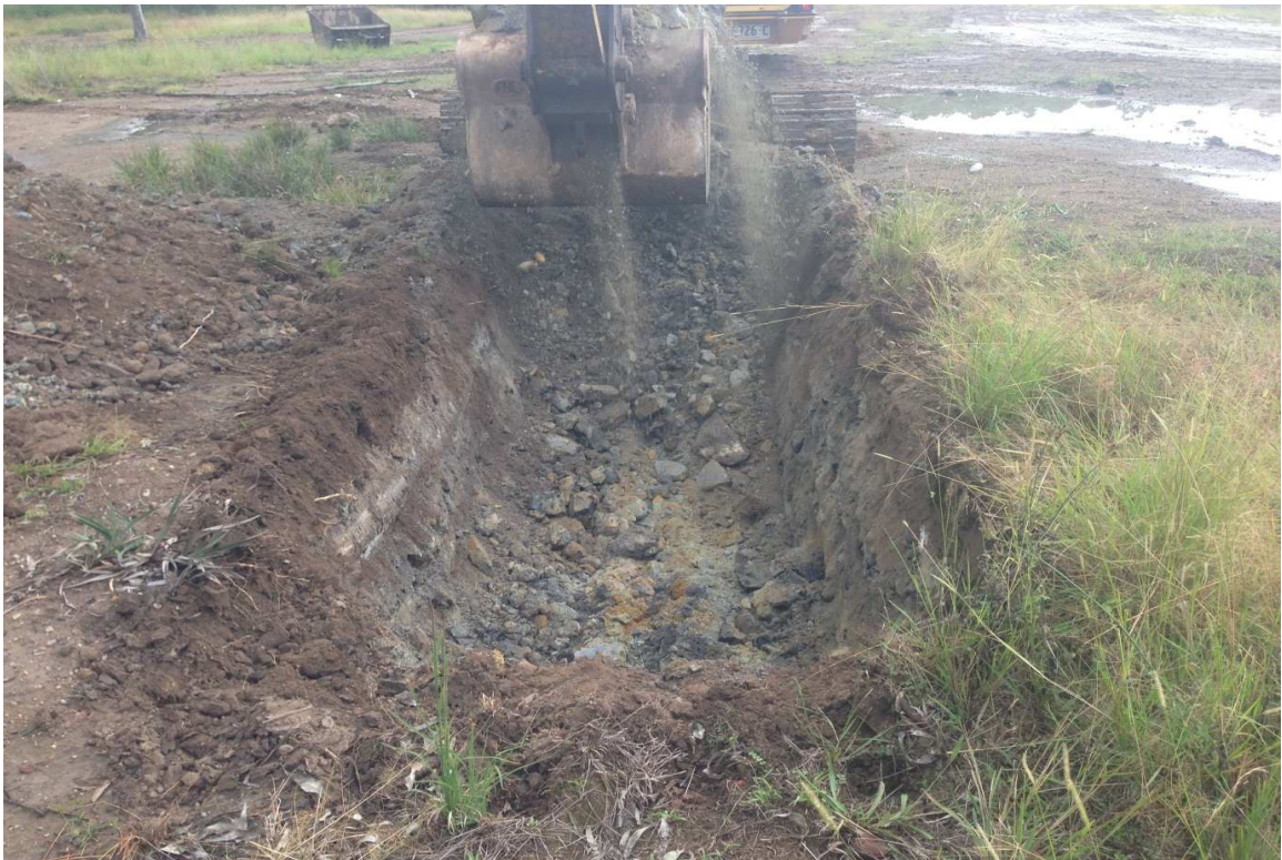
Photograph 2: Excavating test pit TP2 in mining overburden area
