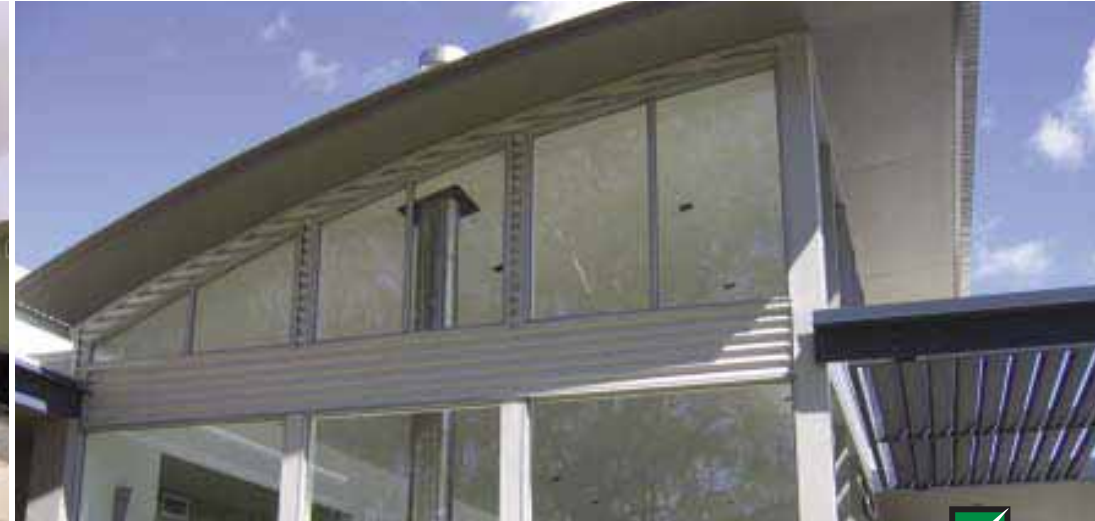
Clear glazing extended to the eaves enhances views.
