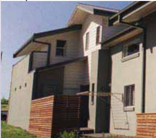
This home has used timber screening to hide utilities from public view
