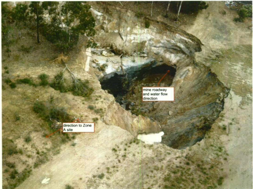
Photo 1: Aerial view of 2007 sinkhole, looking south
