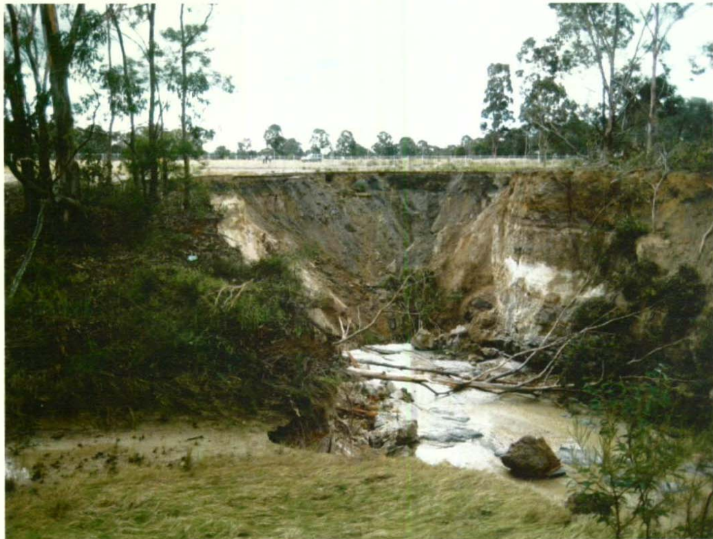
Photo 2: View from Black Creek towards the 2007 sinkhole
