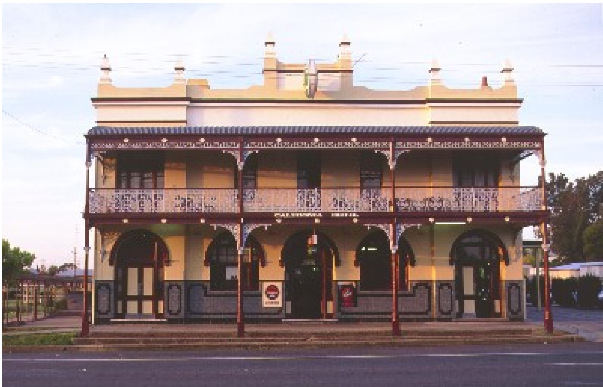
The Caledonia Hotel, Aberdare. Colour schemes which compliment the style of the building will enhance the character of the surrounding area.
