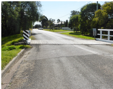
GB17 - The bridge on Anvil Street is a potential hazard for children cycling on road
