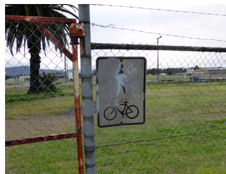
C13 - Shared path signage at the start of the path
