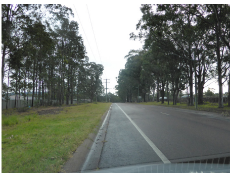
C15 - A narrow, unmarked shoulder for cycling near the intersection of Oakey Creek Road
