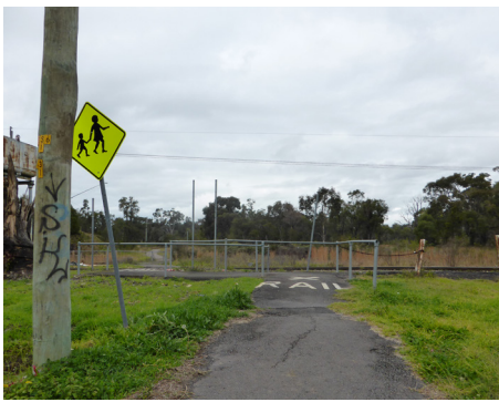
WA13 - The start of the path on Scott Street is currently signed for pedestrians only
