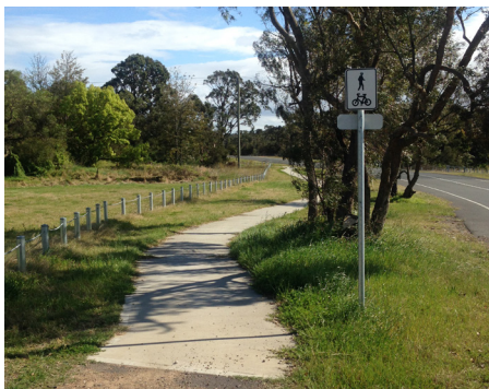
KK16 - The shared path ends on Colliery Street in Stanford Merthyr
