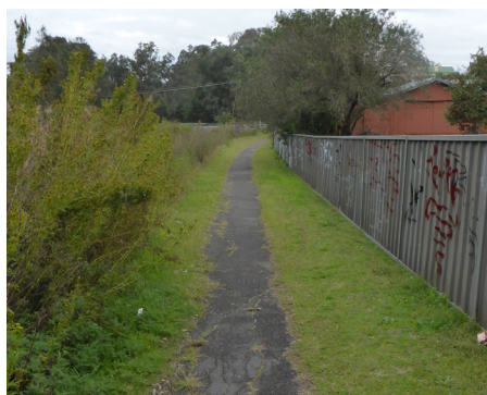
WA11 - The path runs between the side of a property and a small creek
