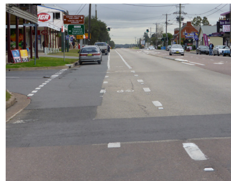
GB08 - On-road lanes exist on both sides of the road through the busiest part of Branxton
