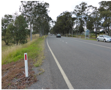
P08 - The road shoulder nearly disappears at this intersection
