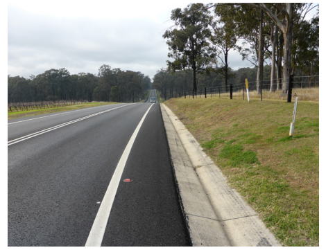
P09 - Some parts of the western section of Broke Road have narrow shoulders
