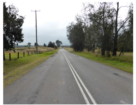
P12 - The final section of the road has no shoulder at all
