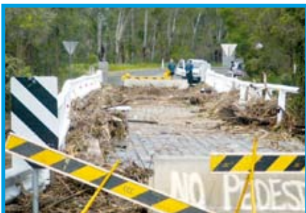
Whitebridge Road Bridge, Mulbring is still closed. A middle pylon was moved by the force of the water.
