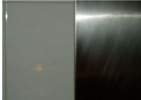
Picture 12: Stainless steel splashback sealed to a tiled wall surface.
