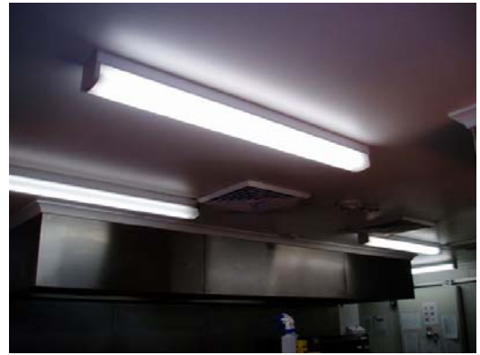
Picture 4: Light fitting flush to ceiling
