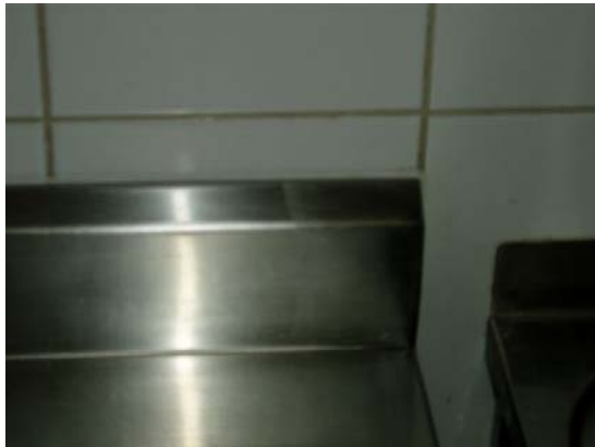
Picture 11: Sealing bench tops to wall.
