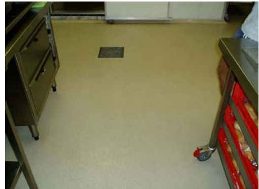
Picture 2: Floor waste
